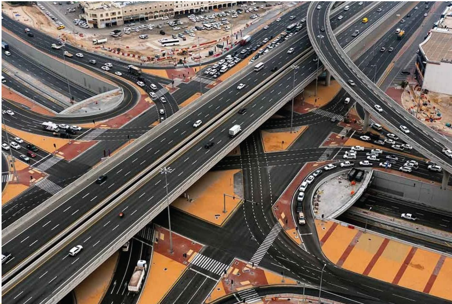
MUBAIREK BRIDGE DOHA, QATAR
